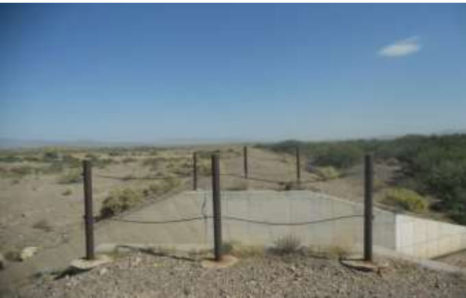
5.b) Medium size structures in upland side channels (for example Halfway detention dam in the photograph)
