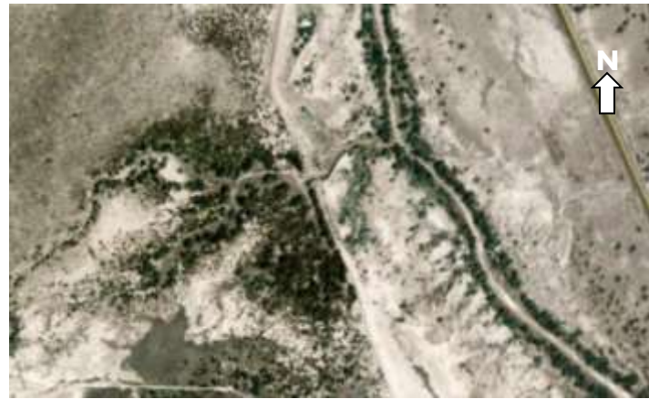
5.a) Ryan dike, viewed from air
